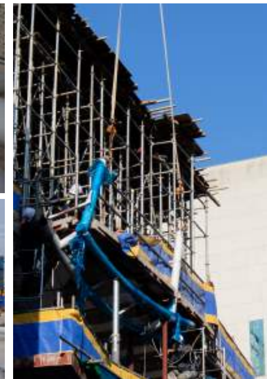
|| Glainno factory in Jisan and Construction site in Seoul. 2018.12.
